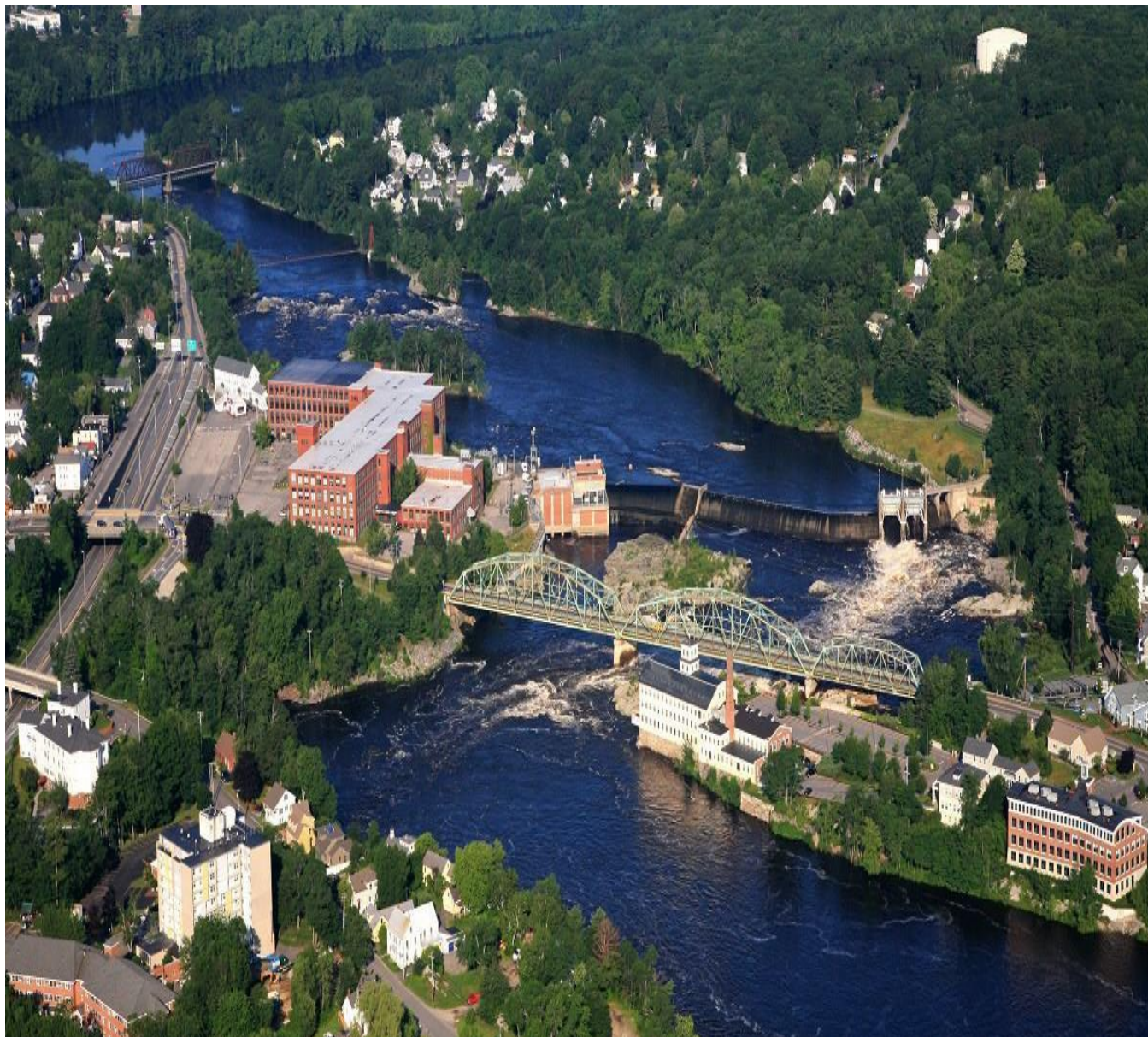
Figure 1. The Brunswick-Topsham Hydropower Station located in Brunswick, Maine. The fishway is located on river right just below the powerhouse. The tailrace is also on river right, separated from the larger portion of the spillway and tainter gates, by a retaining wall and Shad Island located just upstream of the route 201 bridge.
