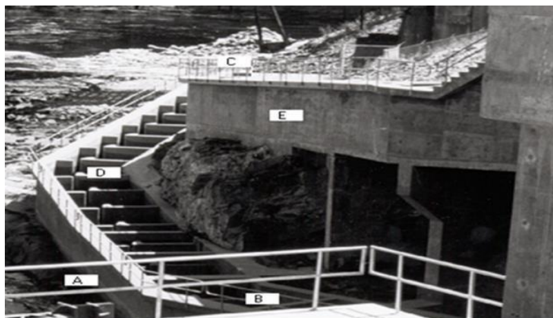
Figure 3. Brunswick fishway; (A) location of river observations, (B) Lower Fishway, (C) Corner Pool, (D) Pool 14, (E) Upper Fishway - Pool 31.
