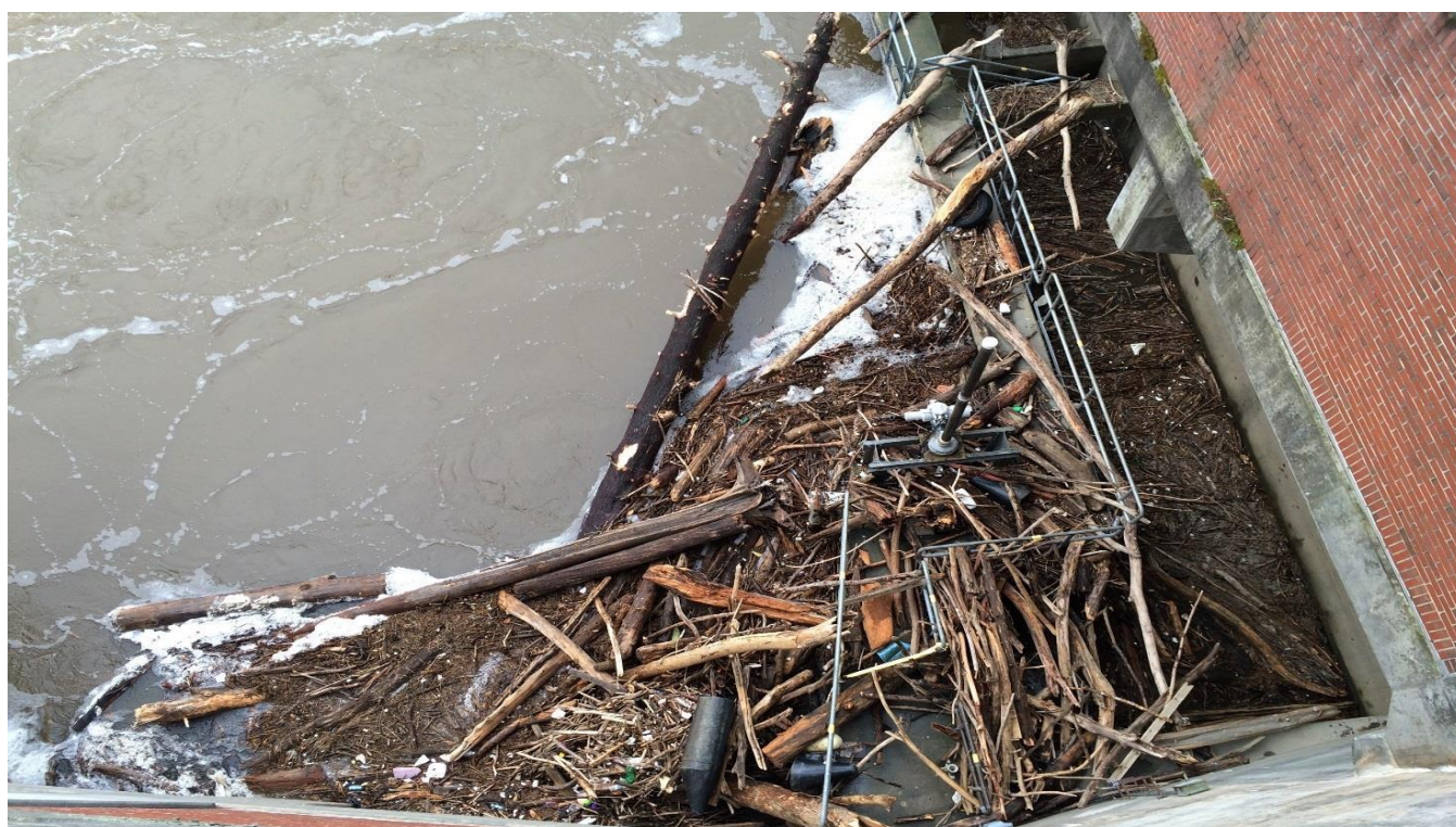
Figure 5. Woody debris blocking fishway entrance caused by high river flows in October resulting in the closure of the fishway on October 30, 2017
